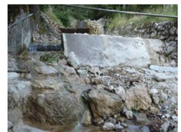
Pictures 22 and 23: Examples of bad practice of water use. Examples show the water abstractions for small hydropower plants on weirs. Downstream of the weirs, only the minimum discharge is left in the bed. Photo: FRIS.
