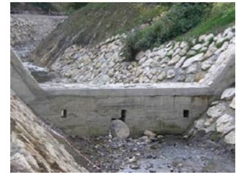
Pictures 18 and 19: Examples of check dams, that disable fish migration. The pictures also shows bank river channelization and bank stabilization with rocks and concrete. Photo: FRIS.
