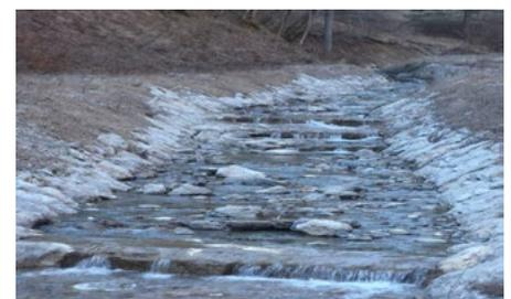
Picture 14 and 15: Examples of stream regulations in the alpine region, inappropriate for fish. The riverbed was widened and straightened, river banks revetment was made with concrete and rocks, riparian vegetation was removed. Photos: FRIS.
