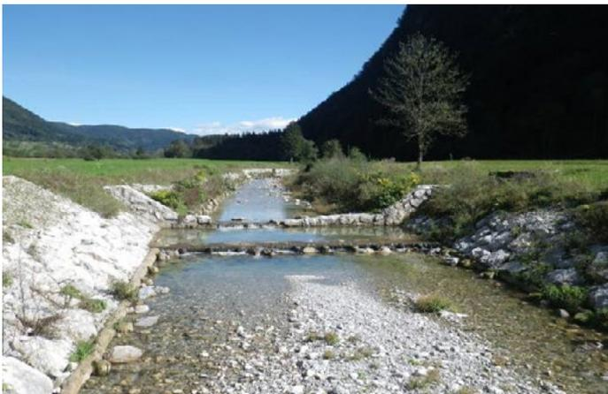
*Picture 12: The channelled section of Ribnica river. The stream is widened, the banks stabilized. Photo: FRIS.*
