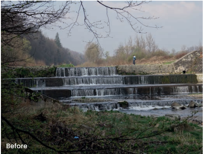
Left: Cascade across the Krzczonówka tributary before it was decommissioned. It was impossible for fish to get to their spawning grounds upstream, and difficult for terrestrial animals to find a safe path along the stream.
