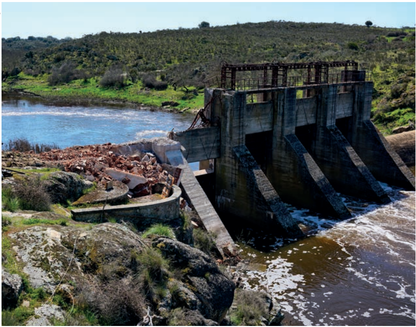
Removal of the 22m-high Yecla de Yeltes Dam on the Huebra River.
