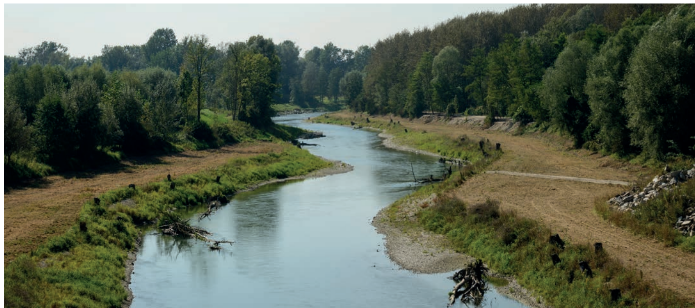
The new bypass channel is near-natural designed with deep areas (pools), fords and inlets and additional habitats for fishes.
