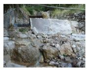
**Pictures 22 and 23:** Examples of bad practice of water use. Examples show the water abstractions for small hydropower plants on weirs. Downstream of the weirs, only the minimum discharge is left in the bed. Photo: FRIS.
