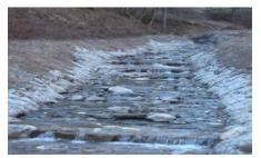
**Picture 14 and 15:** Examples of stream regulations in the alpine region, inappropriate for fish. The riverbed was widened and straightened, river banks revetment was made with concrete and rocks, riparian vegetation was removed. Photos: FRIS.
