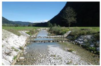
**Picture 12:** The channelised section of Ribnica river. The stream is widened, the banks stabilized. Photo: FRIS.
