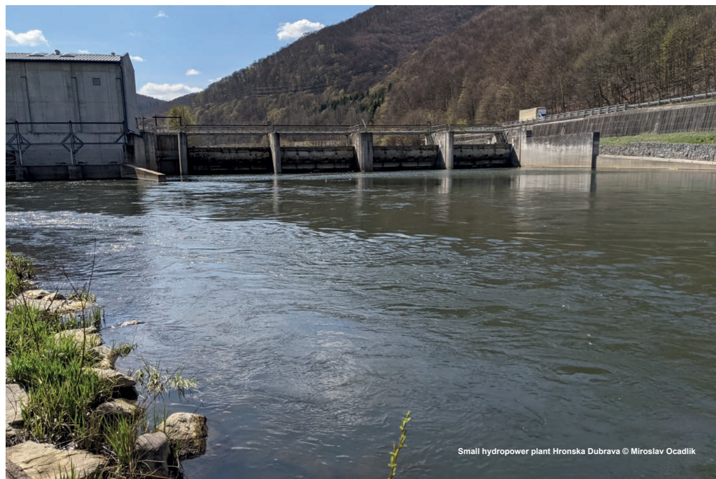
Figure 13: Small hydropower plant Hronská Dubrava built in 2011 on the Hron river. Although the fish pass was part of the construction, it is not operational. The operation of environmental measures is insufficiently dealt with.
